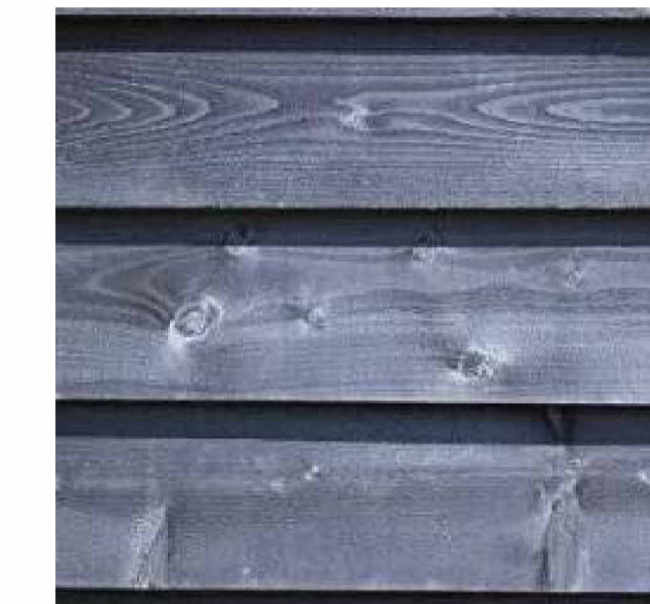
Horizontal Timber Weatherboarding
